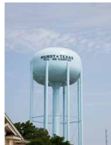
Hurst water tower at TCC NE Campus.
