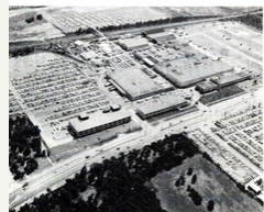
The Hurst Bell Helicopter Plant, shown above, is the world's first that was designed and constructed specifically for the manufacture of rotary-wing aircraft.
